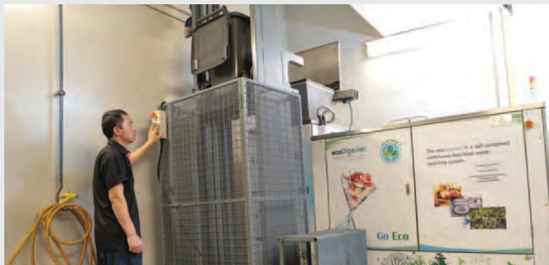
The half-tonne food waste digester handles about 300 kilograms of food waste every day.
