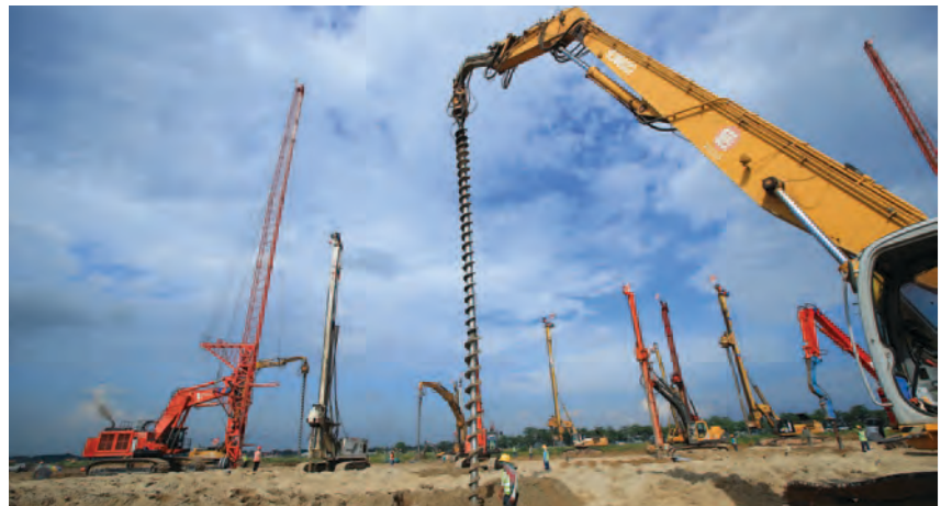
Ground improvement works are being carried out to treat and strengthen the soft marine clay at Changi East.
